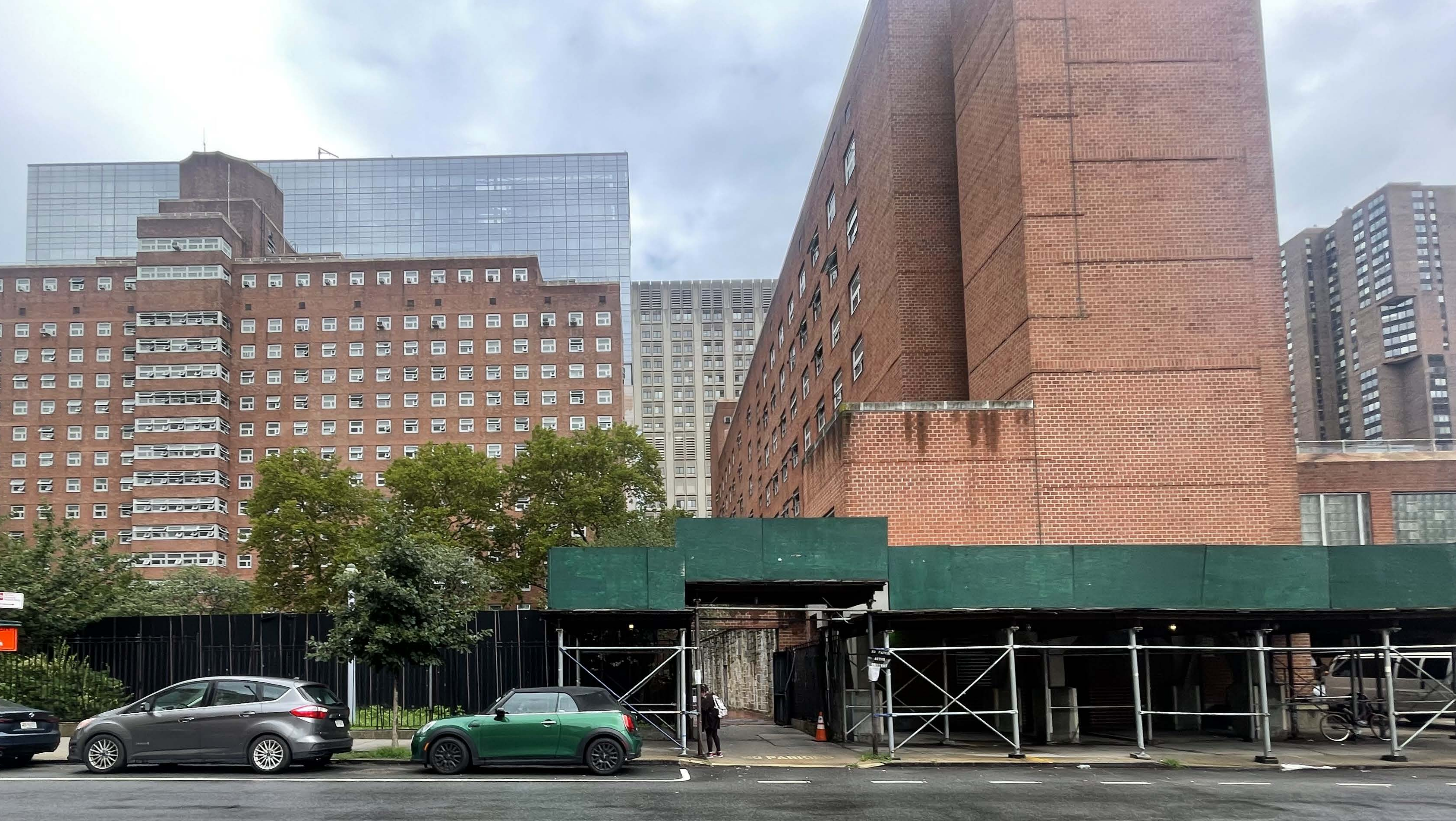
CURRENT VIEW OF THE HUNTER BROOKDALE CAMPUS, MID-BLOCK AT EAST 25TH STREET, LOOKING NORTH
