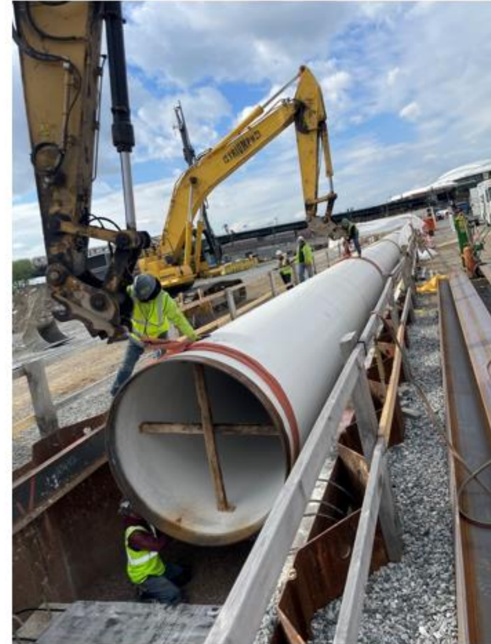
Water main installation
