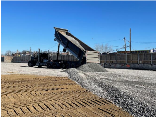
IMPORTING STONE FOR COMPOSITE COVER SYSTEM
