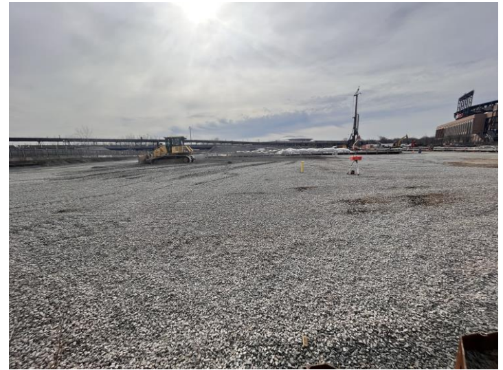
IN-SITU GROUNDWATER TREATMENT AREA RESTORED TO PREVIOUS CONDITIONS
