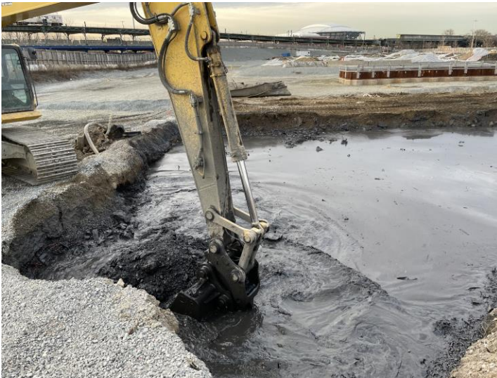
MECHANICAL MIXING OF IN-SITU GROUNDWATER TREATMENT REAGENTS
