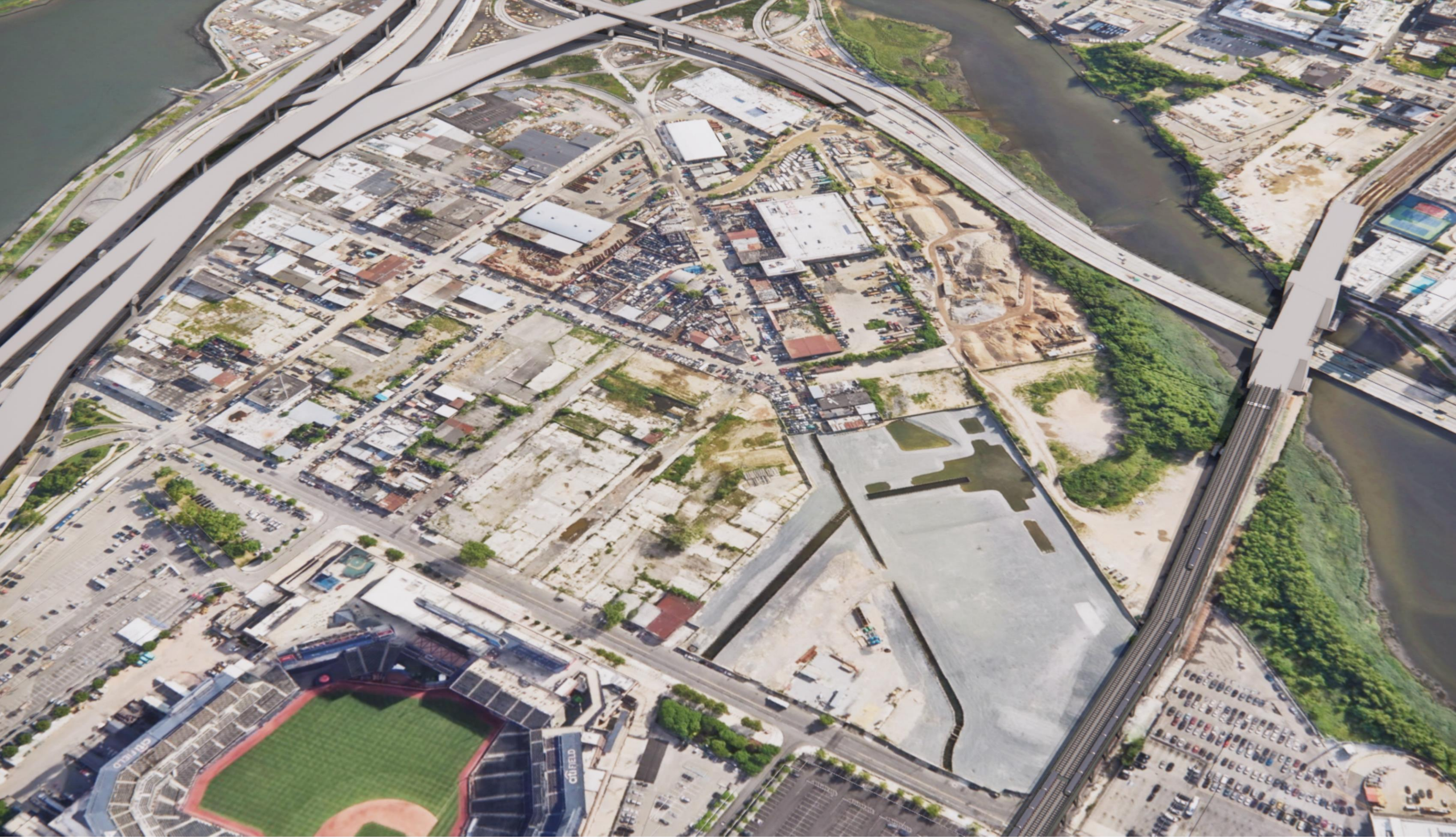
EXISTING CONDITION AERIAL VIEW
