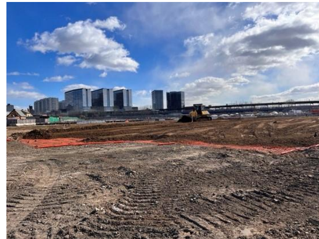
PLACEMENT OF CLEAN FILL FOR COMPOSITE COVER SYSTEM IN AREA F
