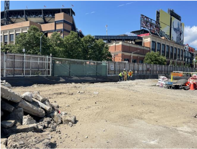
SILT FENCE INSTALLATION AND CONCRETE STOCKPILING
