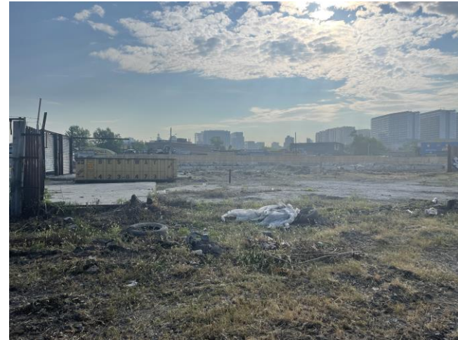
CLEARING AND GRUBBING IN PROCESS
