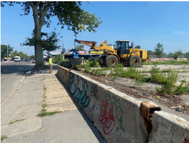
RELOCATING CONCRETE BARRIERS TO THE SIDEWALK ALONG SEAVER WAY
