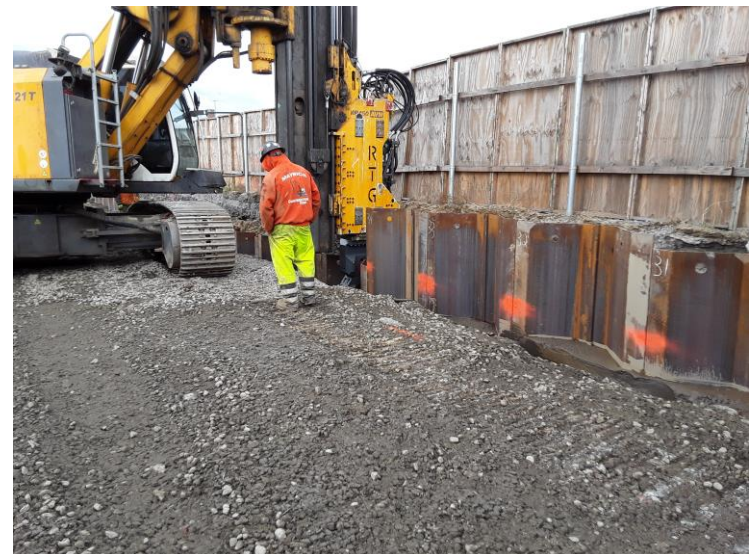
GROUNDWATER CONTAINMENT WALL INSTALLATION
