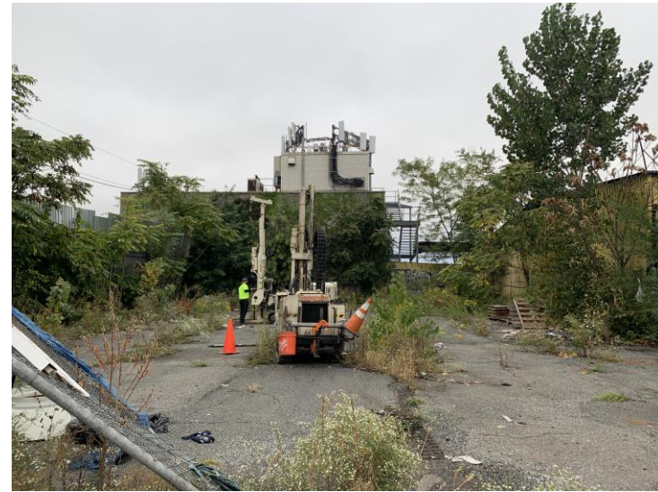
SOIL BORING INSTALLATION
