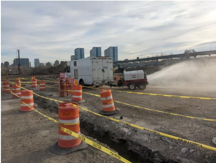
PIPE TRENCHING AND DUST SUPPRESSION
