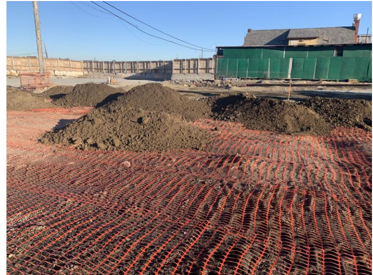
DEMARCATIION BARRIER INSTALLATION POST-SOIL EXCAVATION
