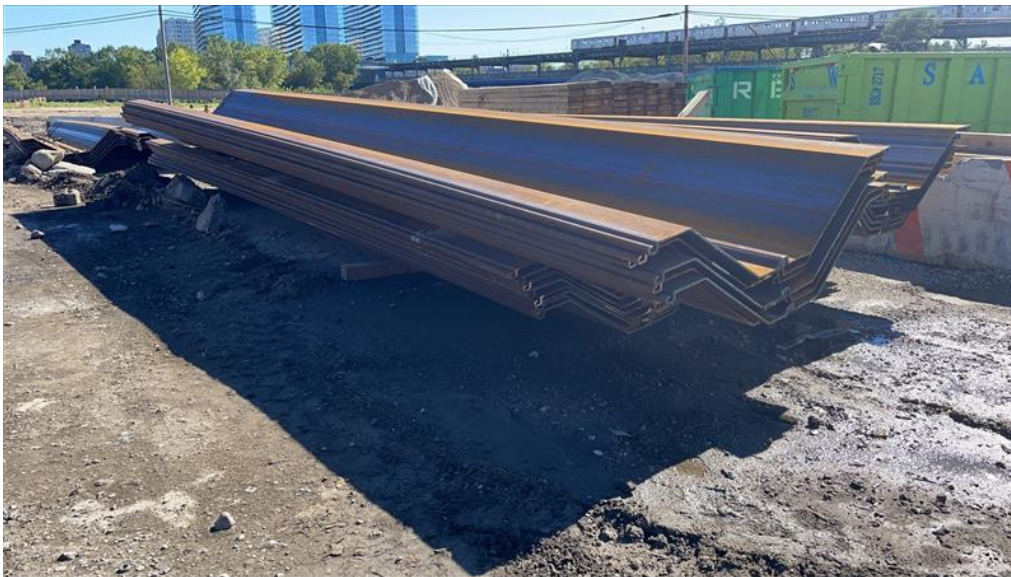
CONTAINMENT CUTOFF WALL SHEETING IMPORTED ONSITE
