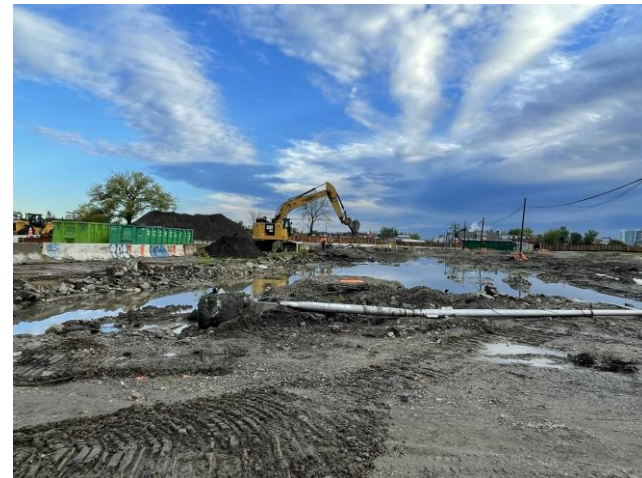
LIGHTPOST DURING REMOVAL
