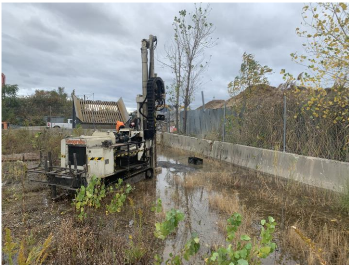
MONITORING WELL INSTALLATION
