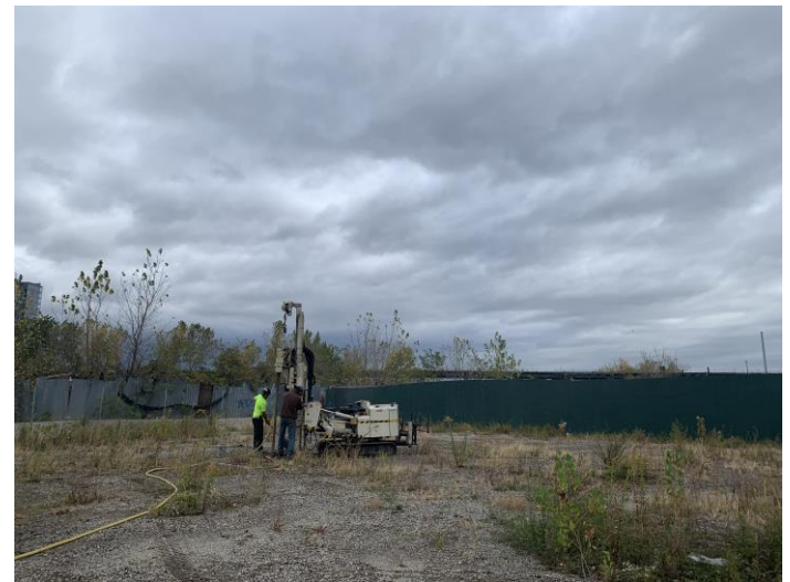
SOIL BORING DRILLING
