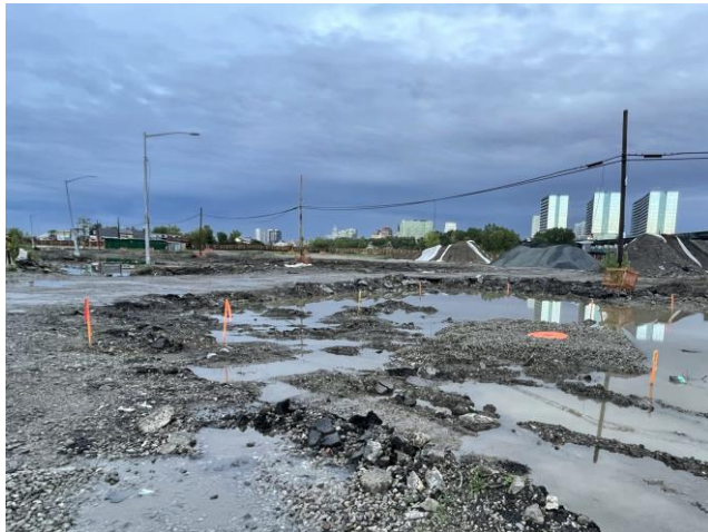
TELEPHONE POLES AND LIGHTPOSTS BEFORE REMOVAL
