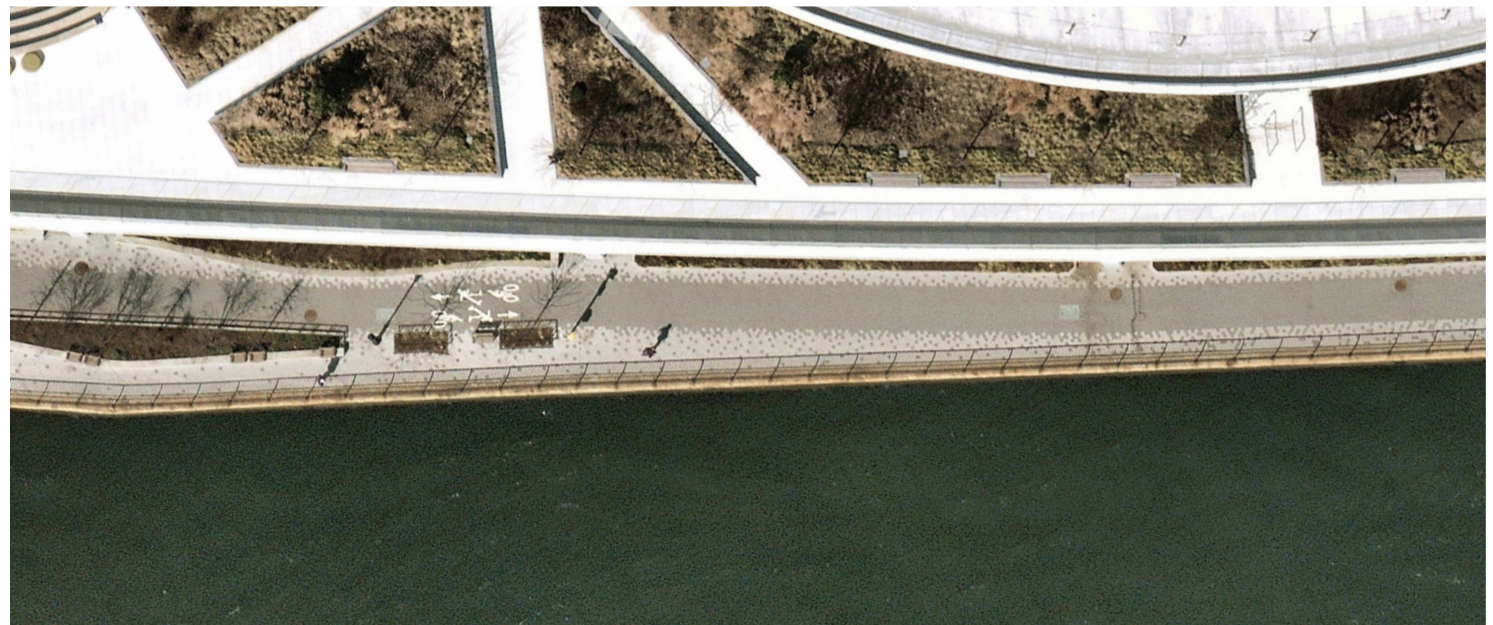
Paver pattern at 68th Street East River Esplanade Reconstruction
