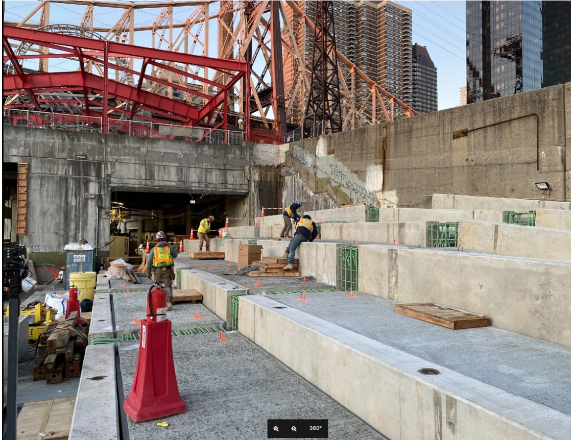
AHG platform construction ongoing
