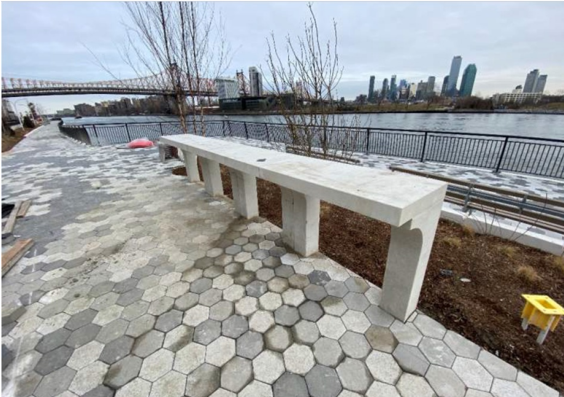
Precast table installed
