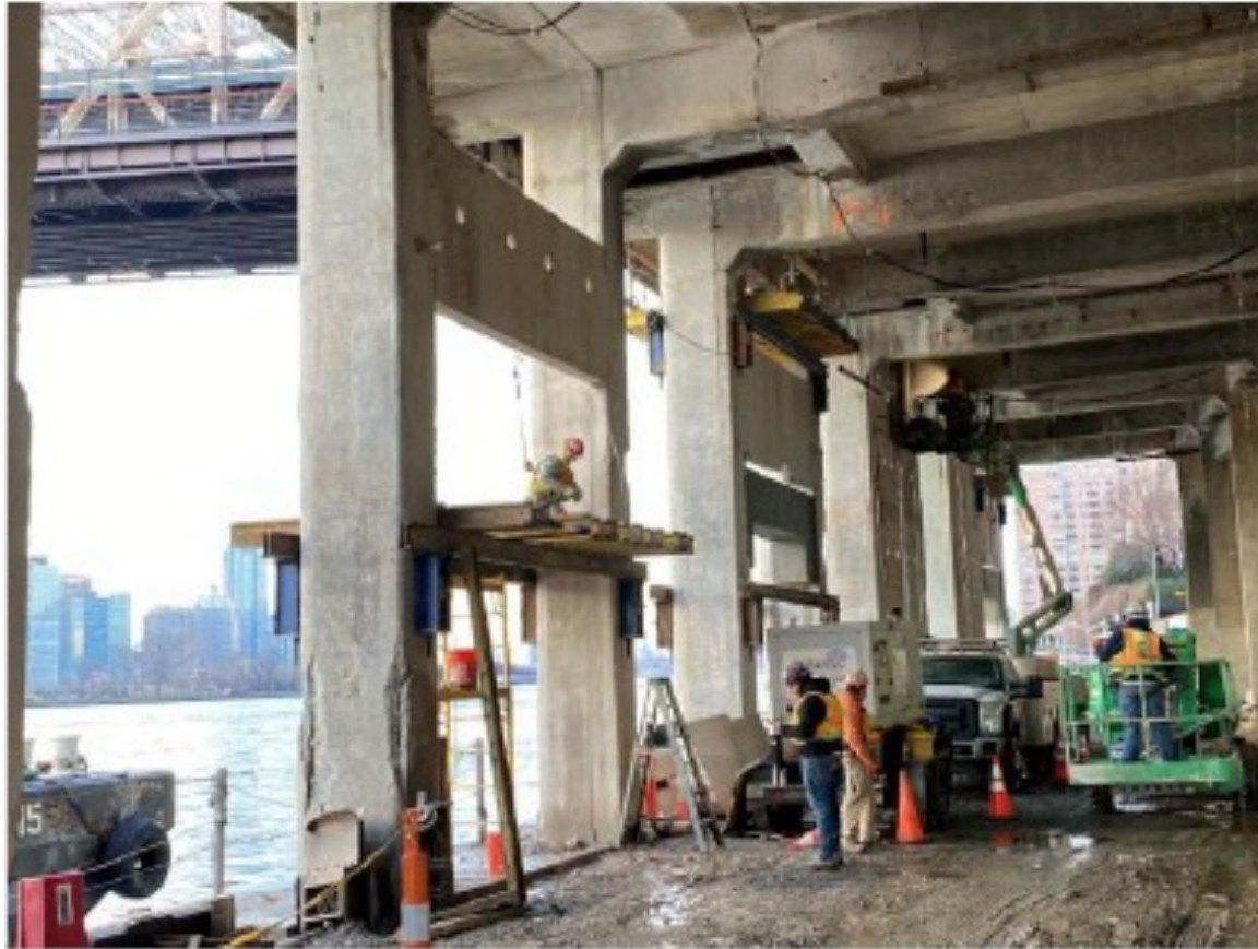
Concrete Curtain Wall removed under the heliport structure
