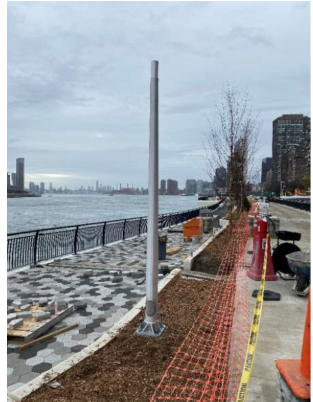
Light poles installed & Planting completed
