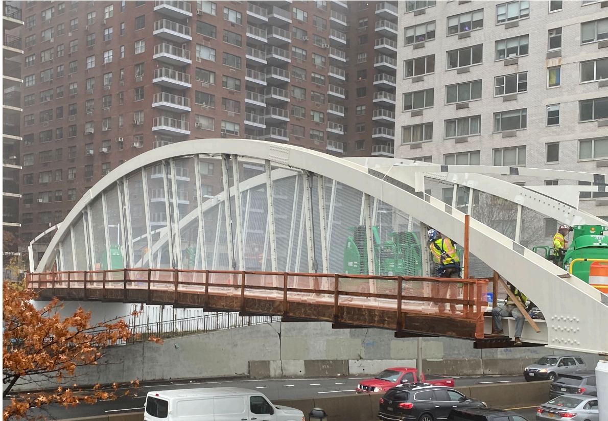
Installation of pedestrian bridge fencing
