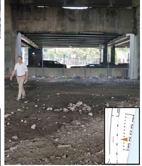
View looking West to FDR
