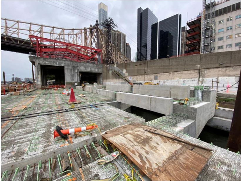
Install Deck Planks
