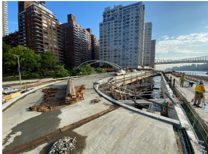
Strip Ramp Edge Forms
