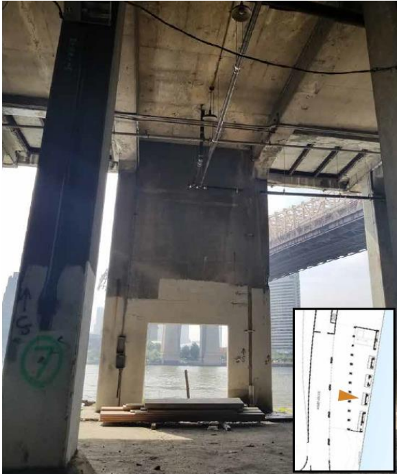
View looking East
