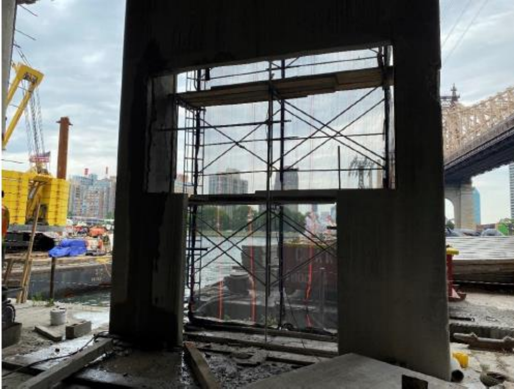
East Curtain Wall Demo
