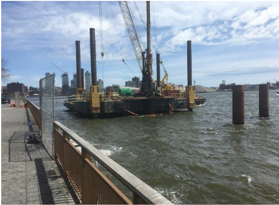
Barge mounted drill rig
