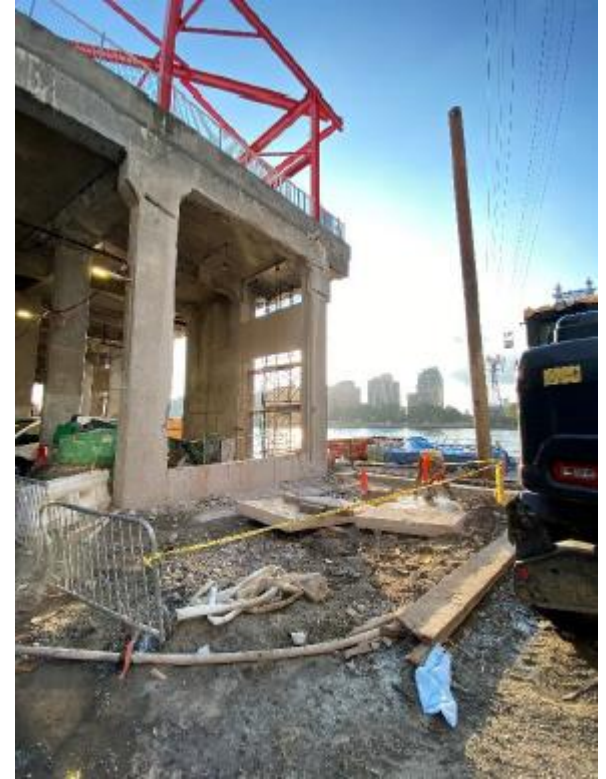
Demo of South Curtain Wall
