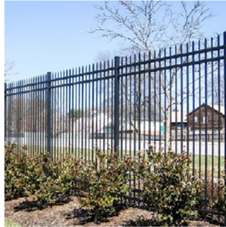
8' Height Black Steel Fence with Vinyl Visual Screen Material: Steel Color: Black
