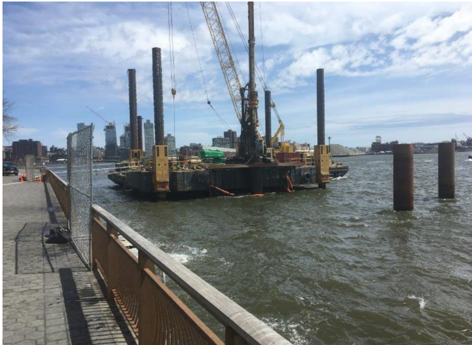
Barge mounted drill rig
