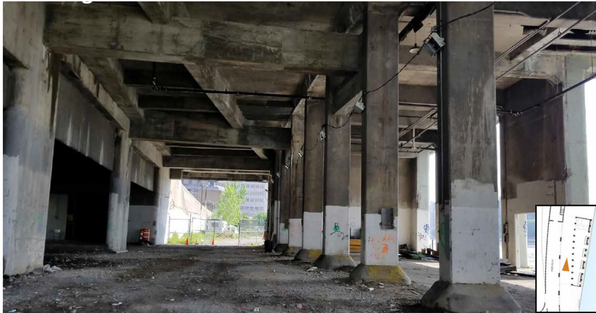
View looking North
