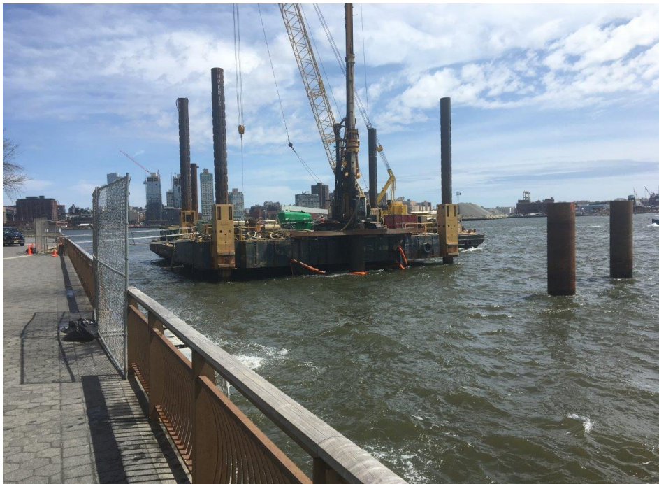
Barge mounted drill rig
