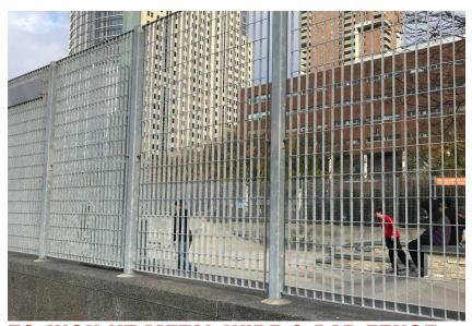
**72-INCH HT METAL WIRE & BAR FENCE** Item: 227 Duffield Fence / **Grigliato Fence / Panel Type E** Manufacturer: Metalco or Approved Equal Material: Galvanized Steel Color / Finish: Galvanized
