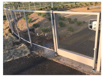
**48-INCH HT** WIRE MESH FENCE + GATES Item: Play Area Fence Manufacturer: Jakob Rope Systems / Cable Railing System Material: Stainless Steel Cable Mesh / Painted Steel Pipe Frame, Color: Silver
