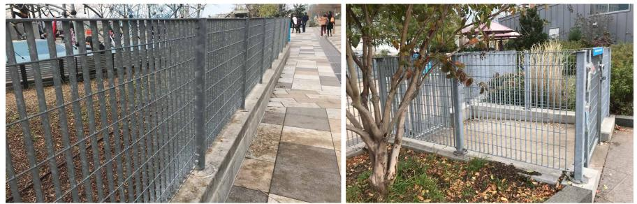
**30-INCH HT // 48-INCH HT METAL WIRE & BAR FENCE + GATES** Item: Dog Park Fence / Grigliato Fence / Panel Type A Manufacturer: Metalco or Approved Equal Material: Galvanized Steel Color / Finish: Galvanized
