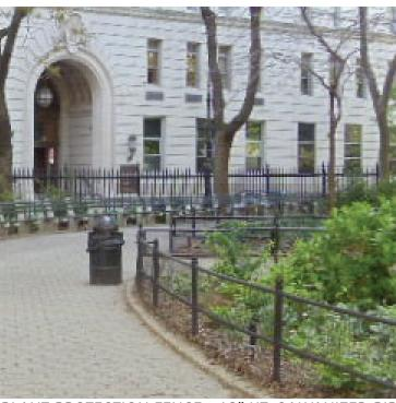
PLANT PROTECTION FENCE - 18" HT. GALVANIZED PIPE RAIL OR COATED STEEL POST
